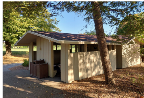
Halfway House renovation
