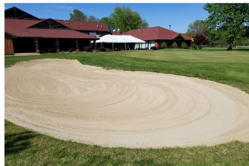
Bunker renovation is nearing completion!
