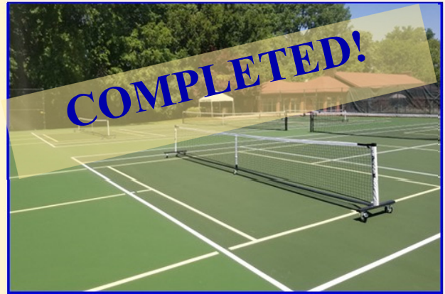
TENNIS / PICKLEBALL COURT RESURFACING
